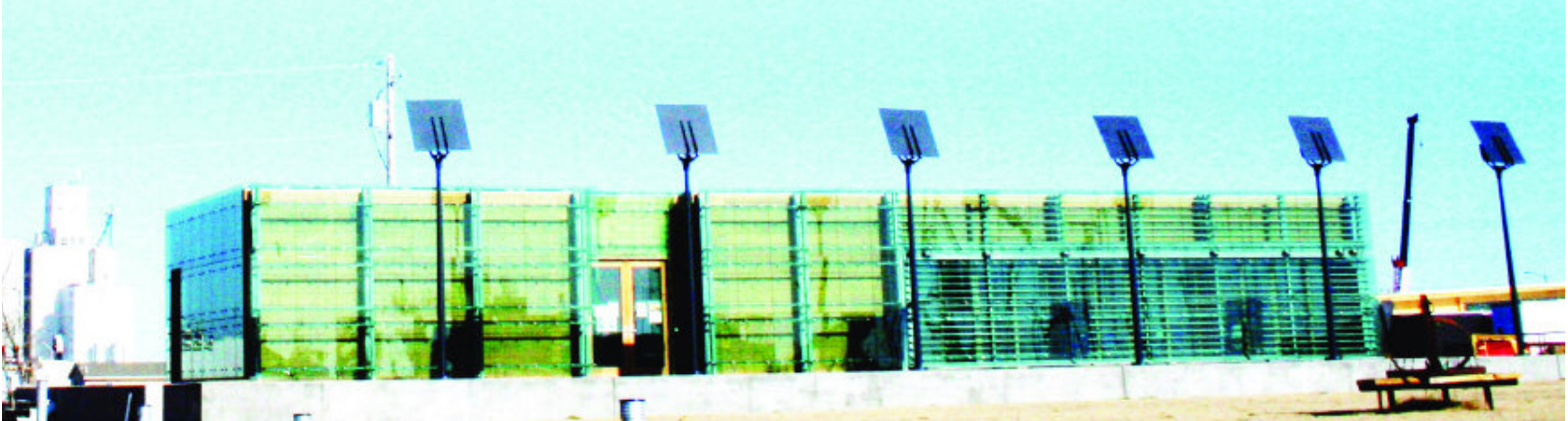
The Arts Center in Greensburg, Kan. is one of many public buildings that have been designed to strict efficiency standards after a tornado destroyed the small town.
